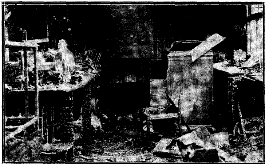
The extent of the damage caused by the fire in Captain Eckersley's wireless station may be clearly seen here. The transmitting valve on the table on the left was the only one of twenty valves to survive.
